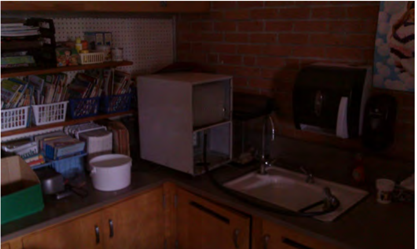
A dehumidifier was draining into the hand washing sink of the Southwest classroom. (Above image)
